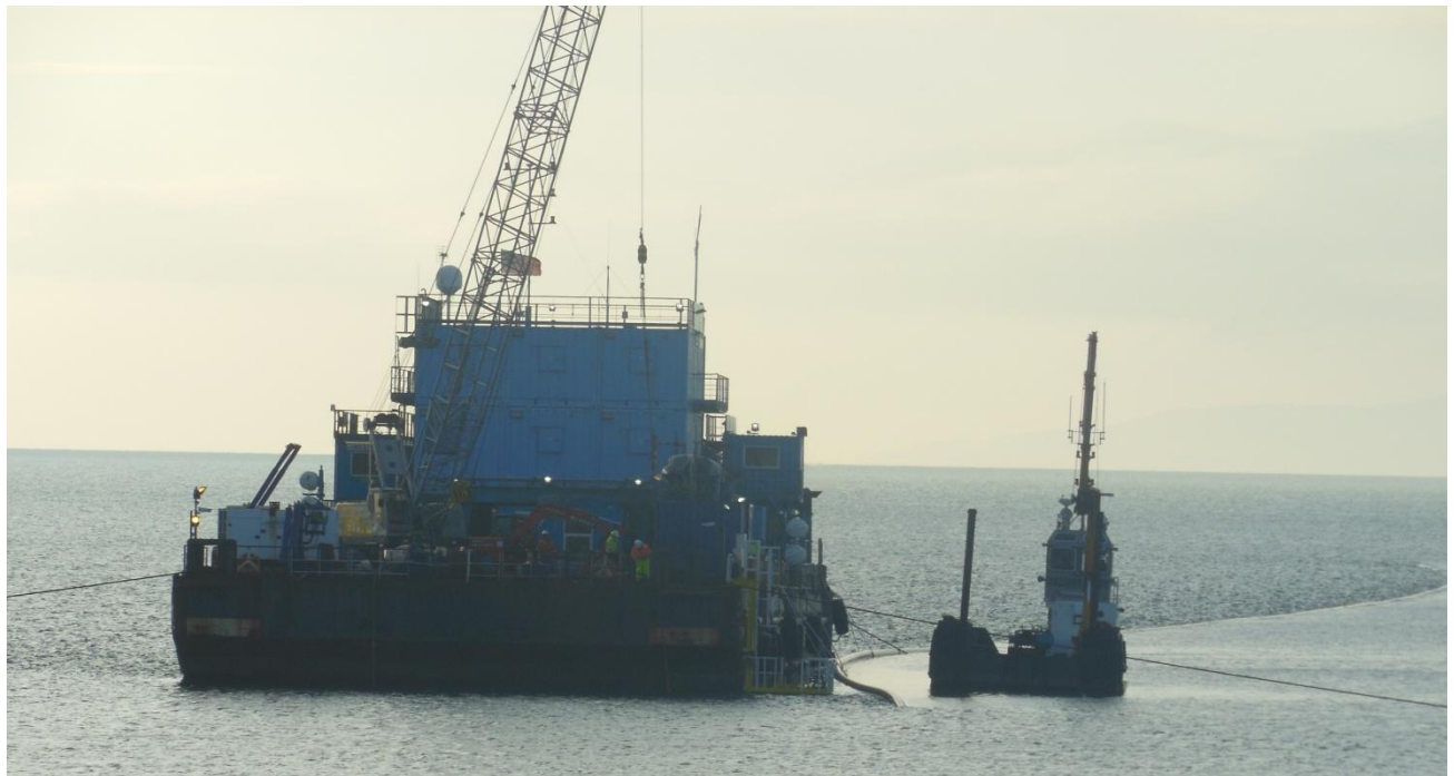
Figure 20. Large barge with four point anchoring and workboat. On the right hand side of the barge the duct can be seen being pulled into the HDD. The water depth is approximately 4m.
