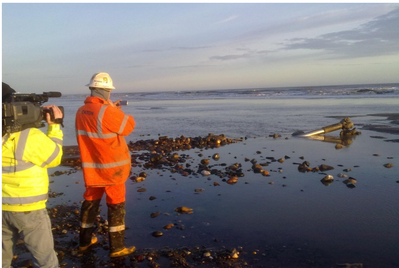
Figure 10. HDD exit on the Humber Gateway project illustrating the short HDD option of exit near MLW.
