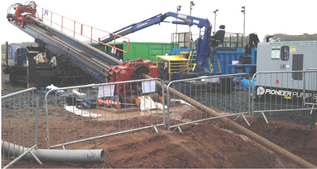
Figure 13. Example HDD rig of similar size to that required for the HDD's.
